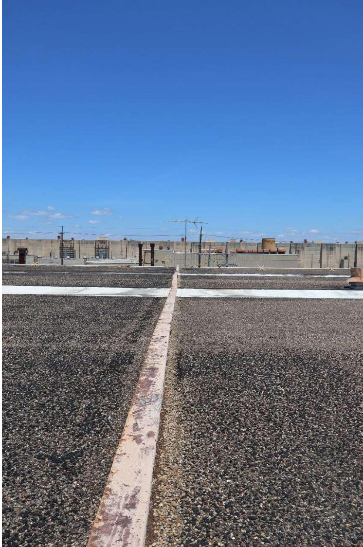
Main High roof – Expansion joint looking North
