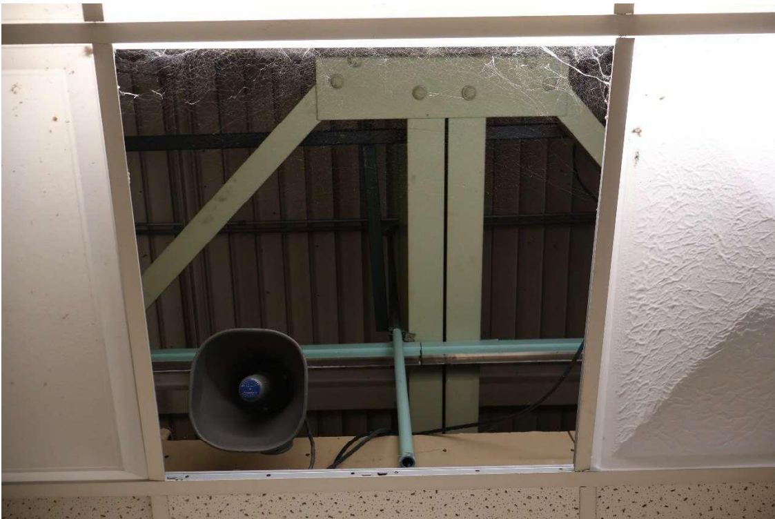
Metal decking on East side of mezzanine
