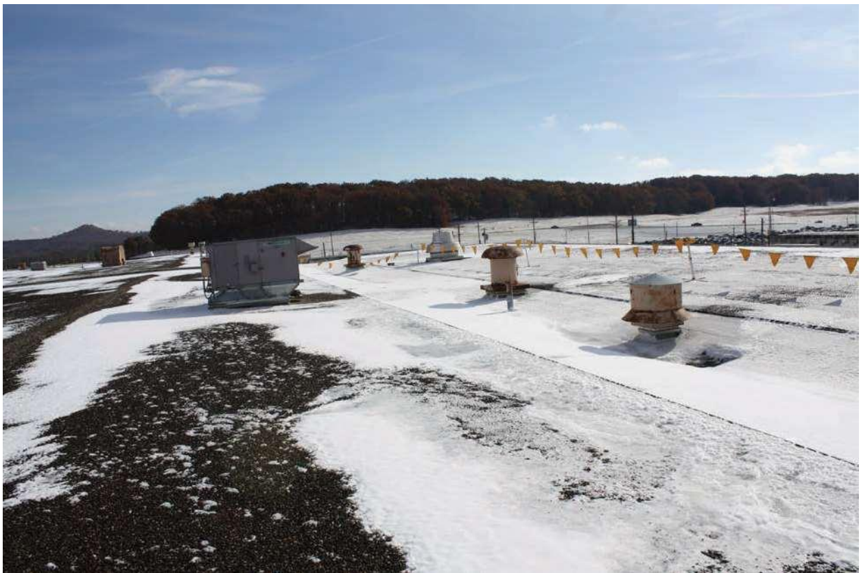
Looking East at TPO Repair of Valley
