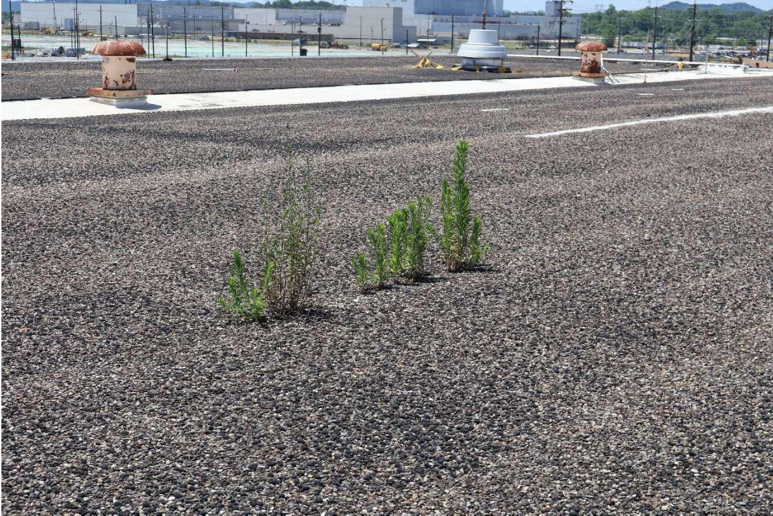
Main High roof – Vegetation
