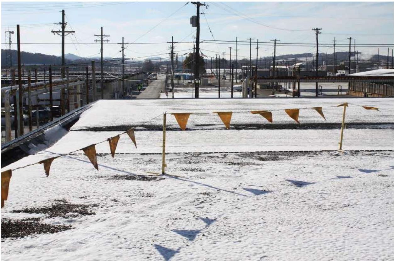
Looking South – Main Low Roof
