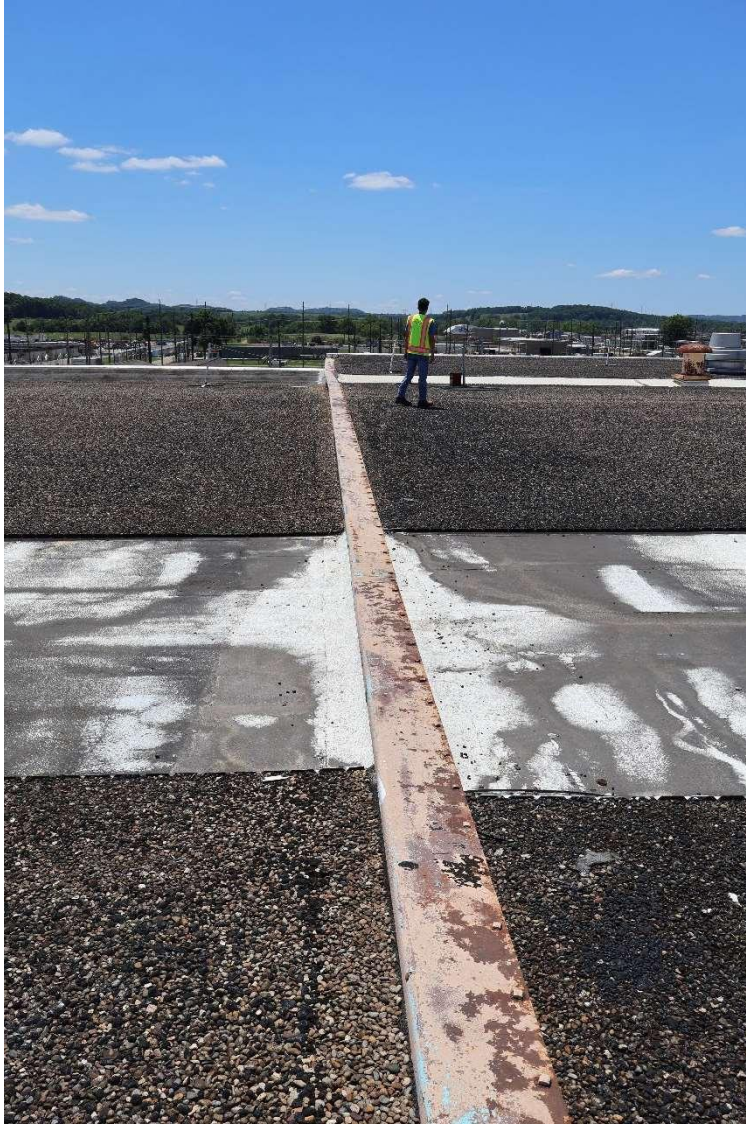
Main High roof – Expansion joint looking South
