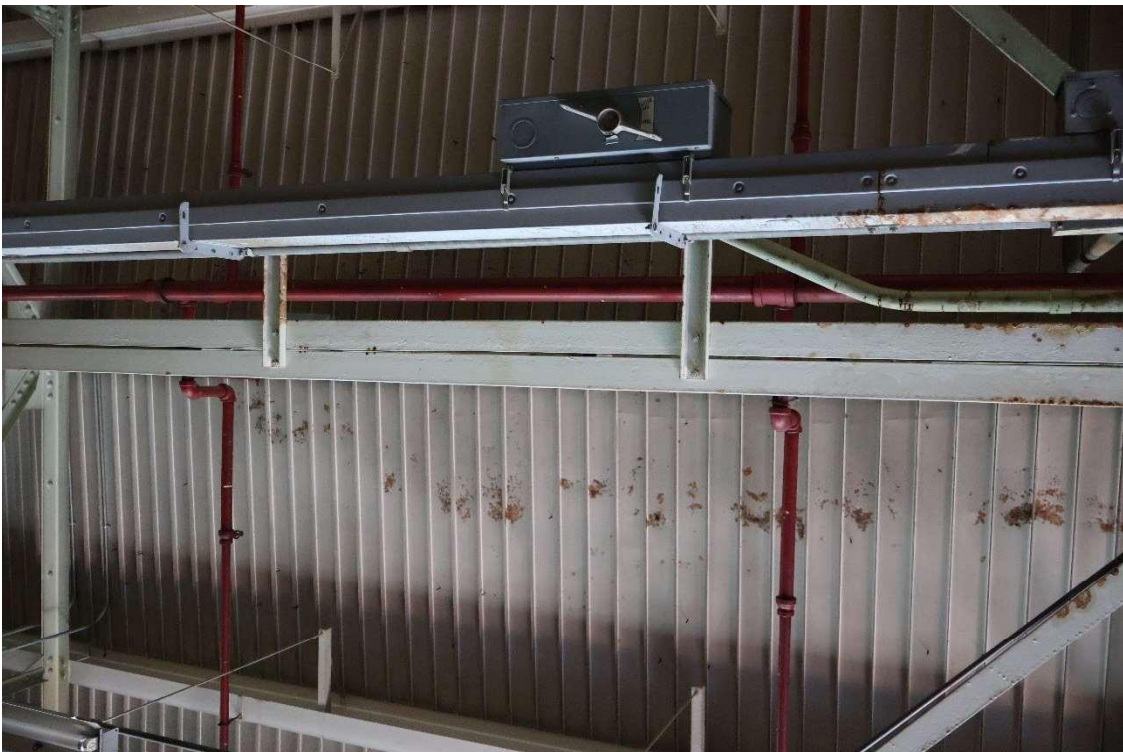
Roof above the picture shown above, at column B13
