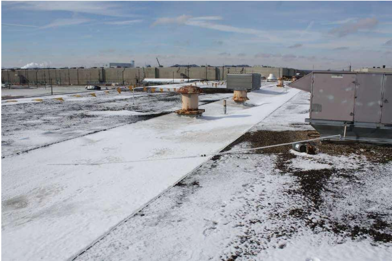
Looking East at TPO Repair of Valley
