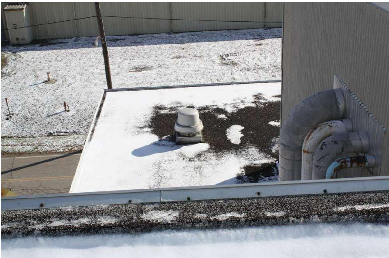
Looking East – Lower Roof of Building Addition (No Physical Walkdown)
