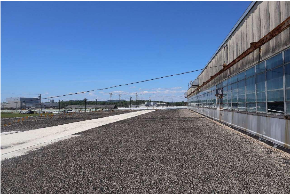
Main Low roof looking West
