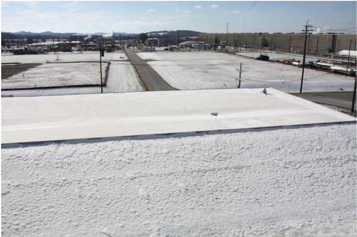
Looking South from Highbay at New TPO on Main Low Roof
