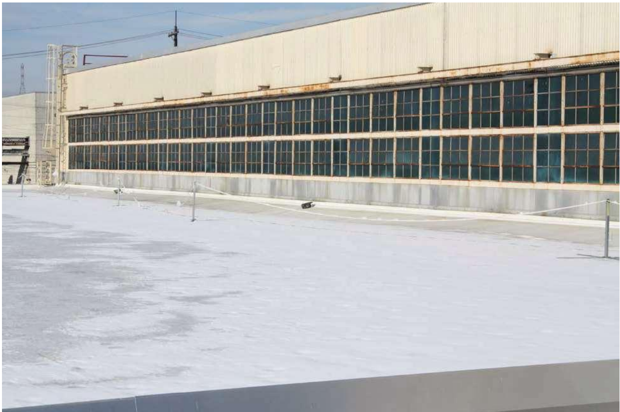
Looking Northwest – New TPO on Main Low Roof
