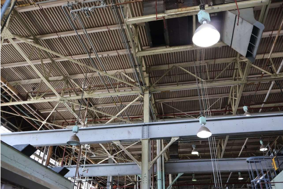
Near column K19
