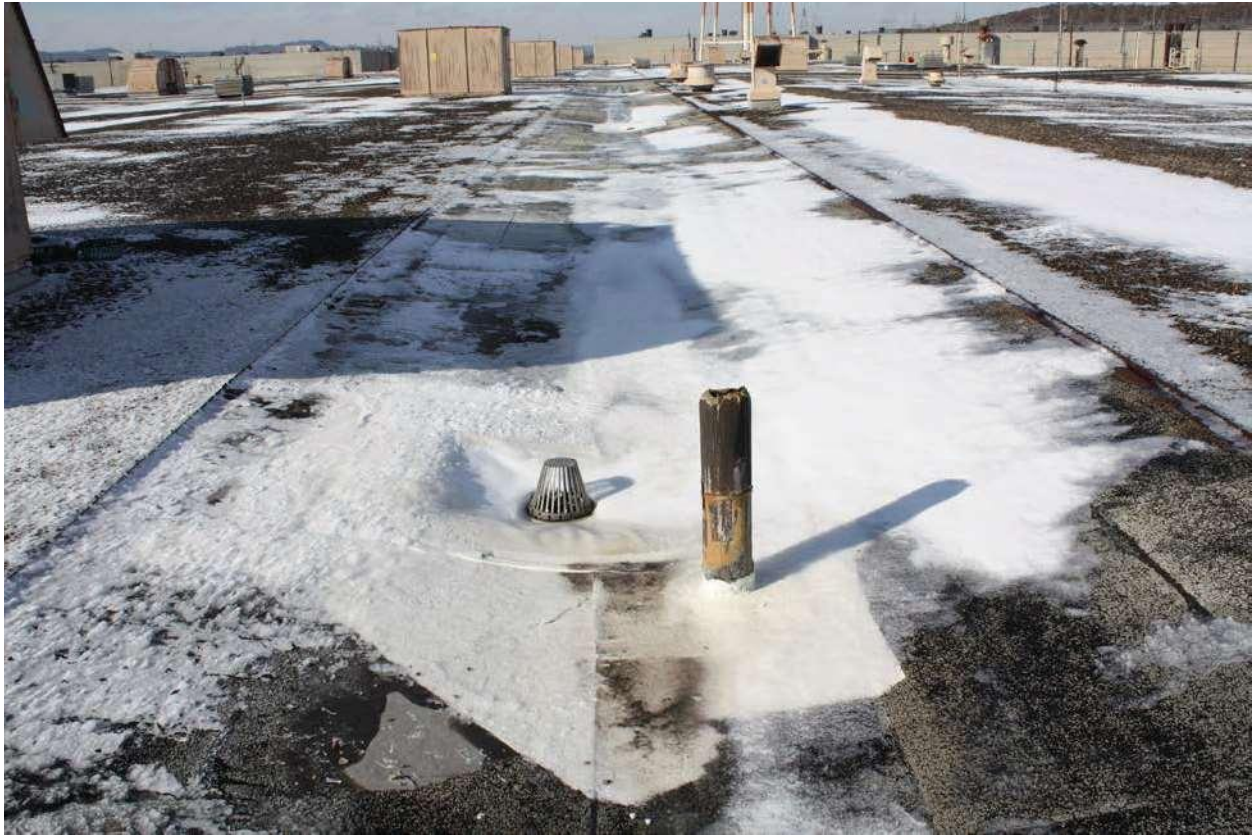
Looking West – Highbay Roof
