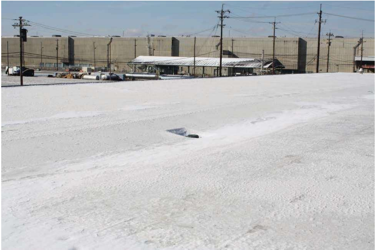
Looking Southwest – New TPO on Main Low Roof
