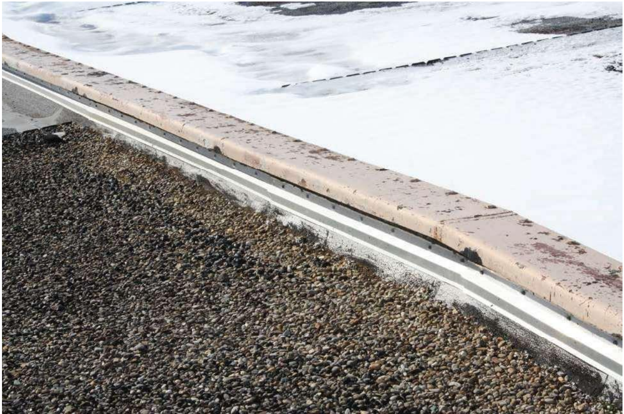
Highbay Expansion Joint, Typical
