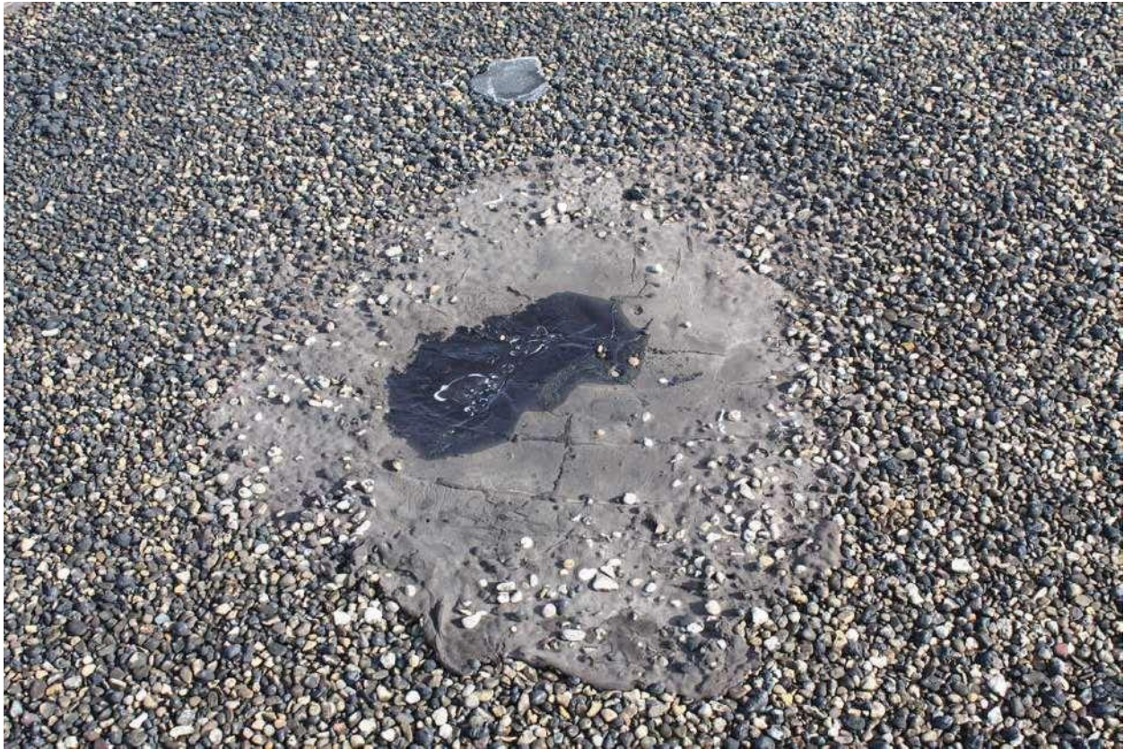
Highbay – Patching of Built-up Roof
