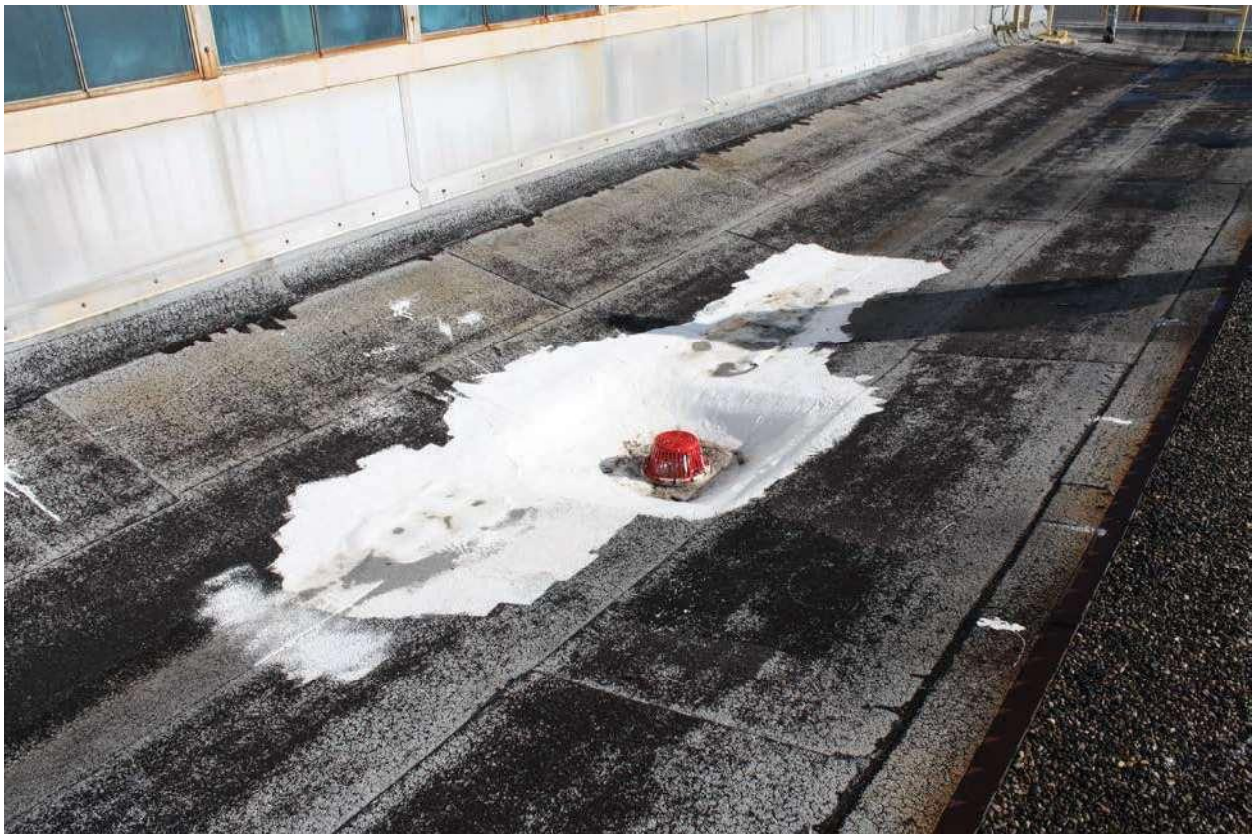
Main Low Roof – Recent Repair of Roof Drain
