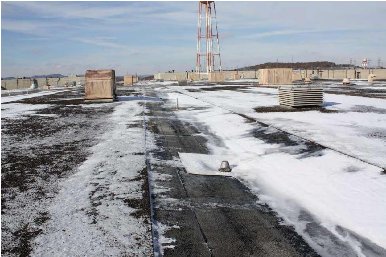
Looking West – Highbay Roof
