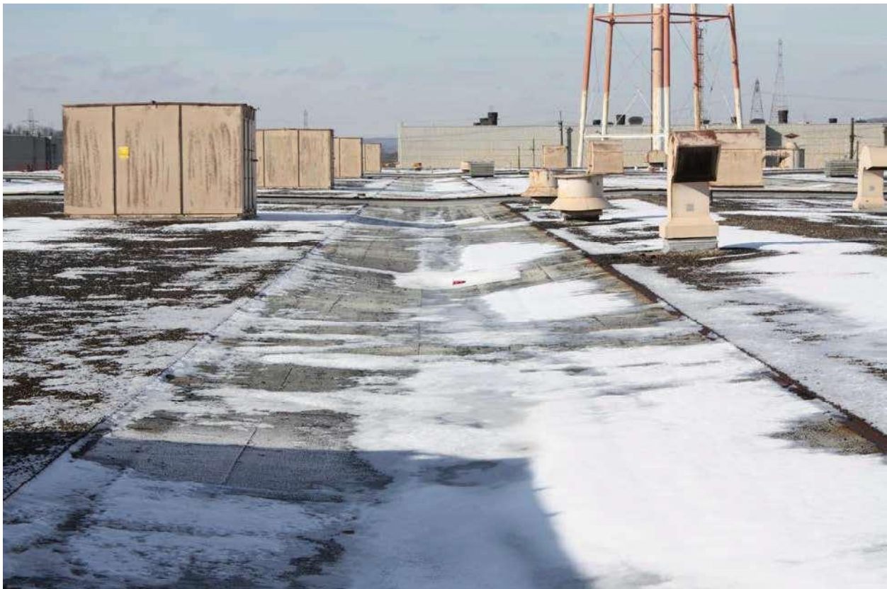
Looking West – Highbay Roof
