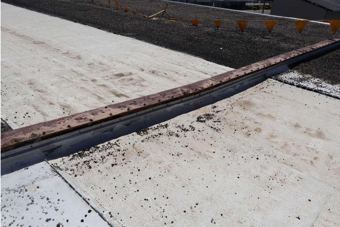
Main Low roof – Expansion Joint
