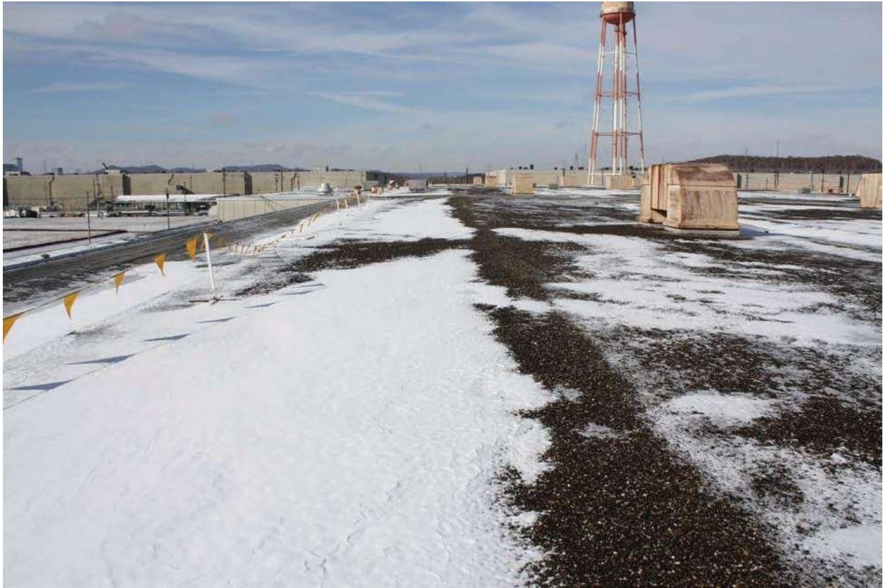
Looking North – Highbay Roof
