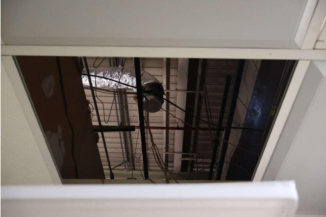
Metal decking near the center of the mezzanine
