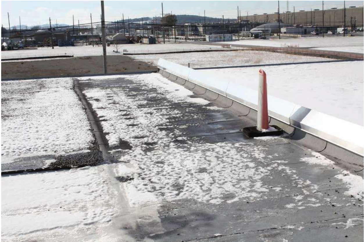
Looking South – Repair at Expansion Joint
