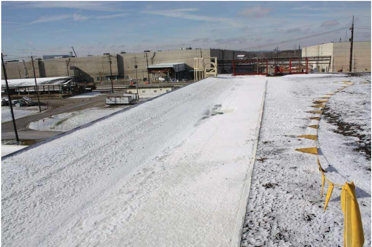
Looking East – New TPO in South Valley
