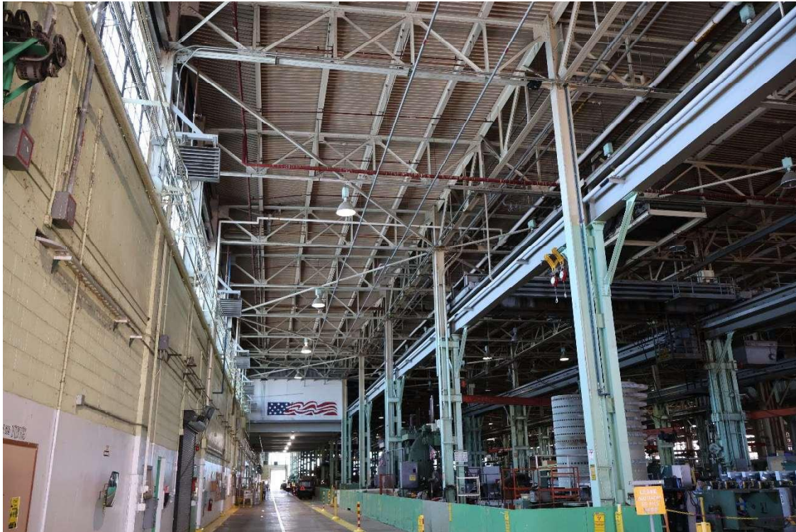
Overall roof, standing near column D20
