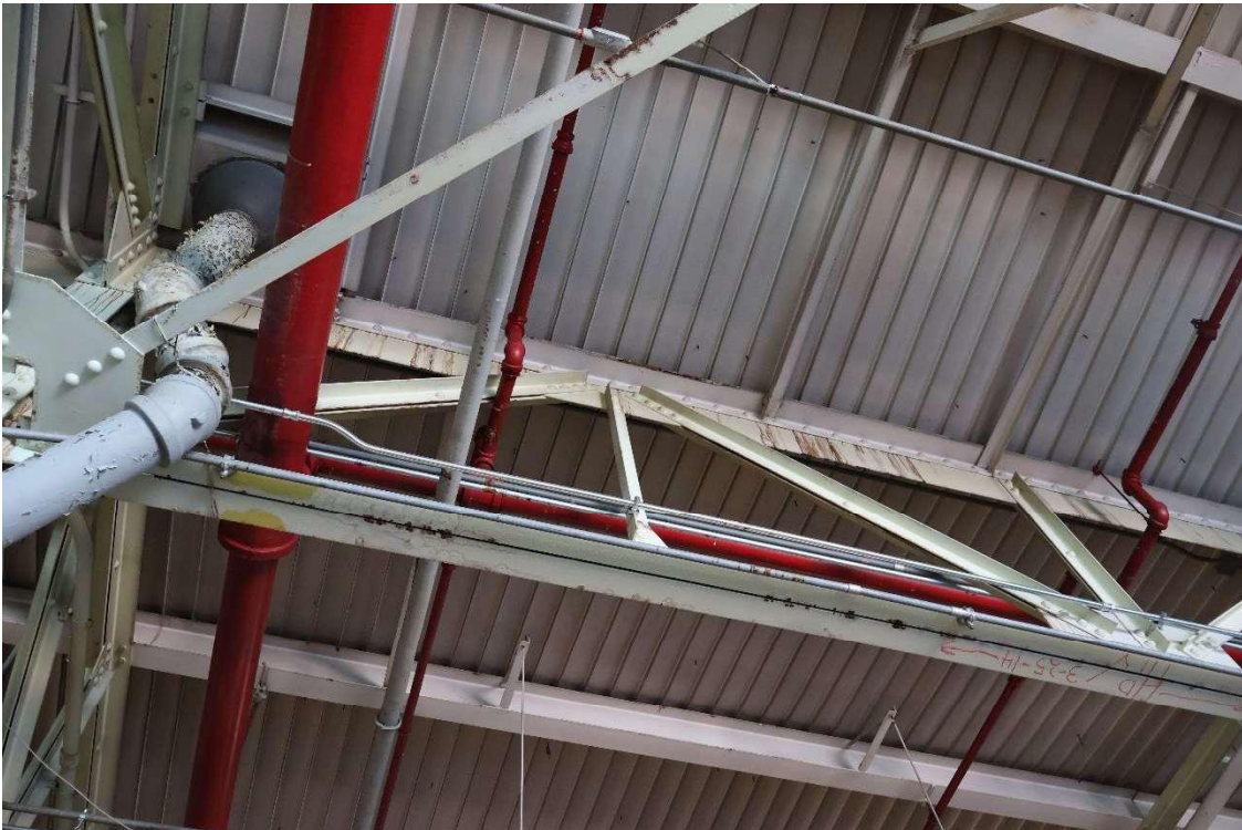
Near column B8
