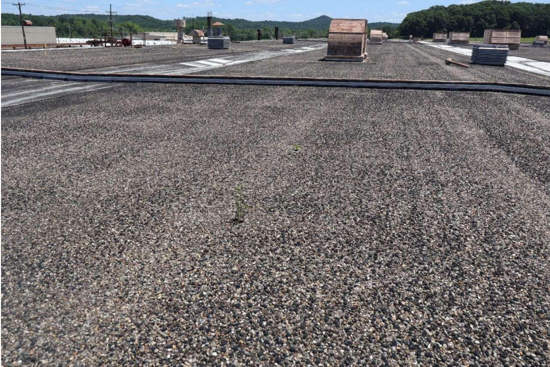
Main High roof – Vegetation
