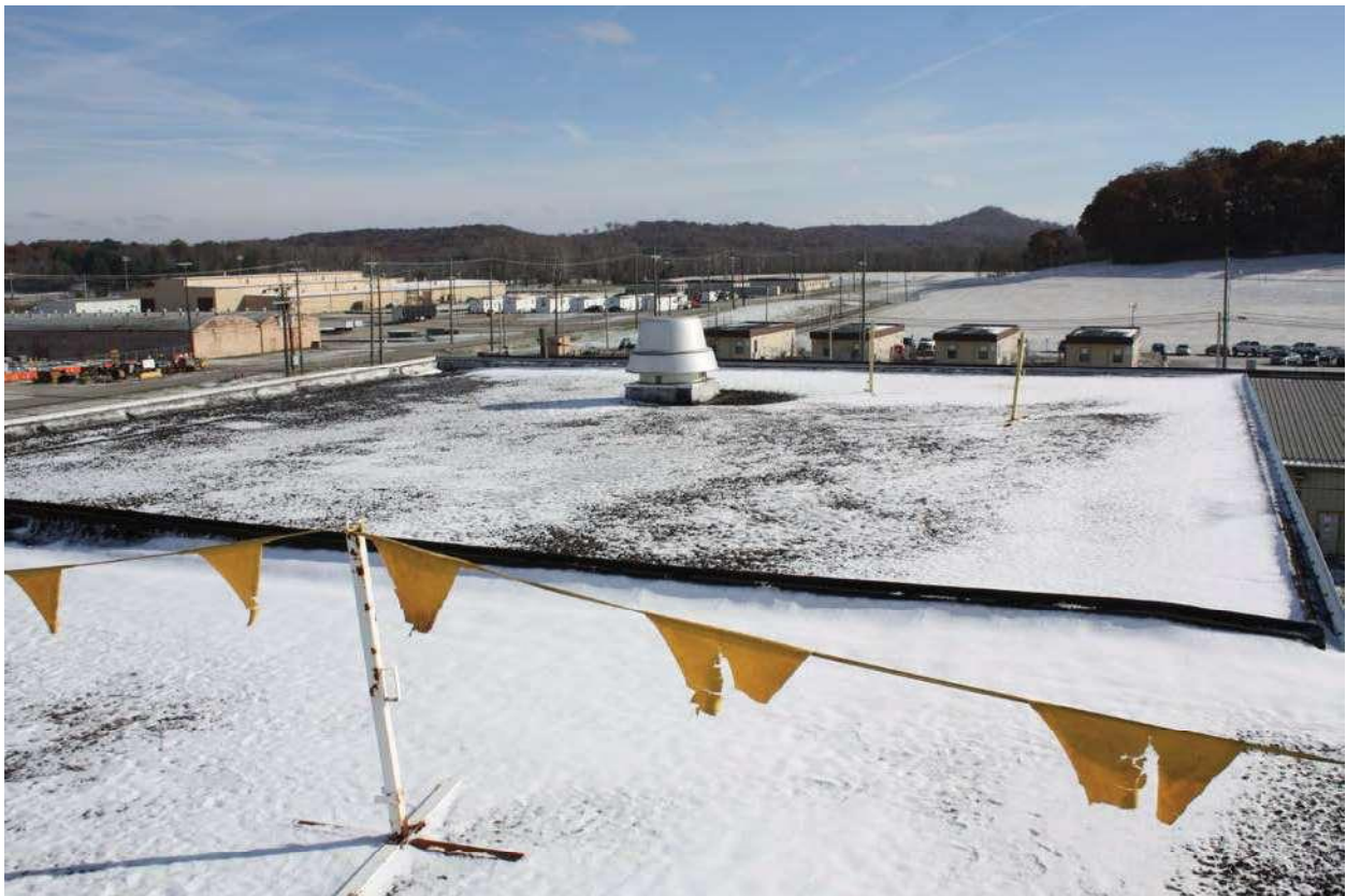
Looking East – Building Addition Roof (No Physically Walkdown)
