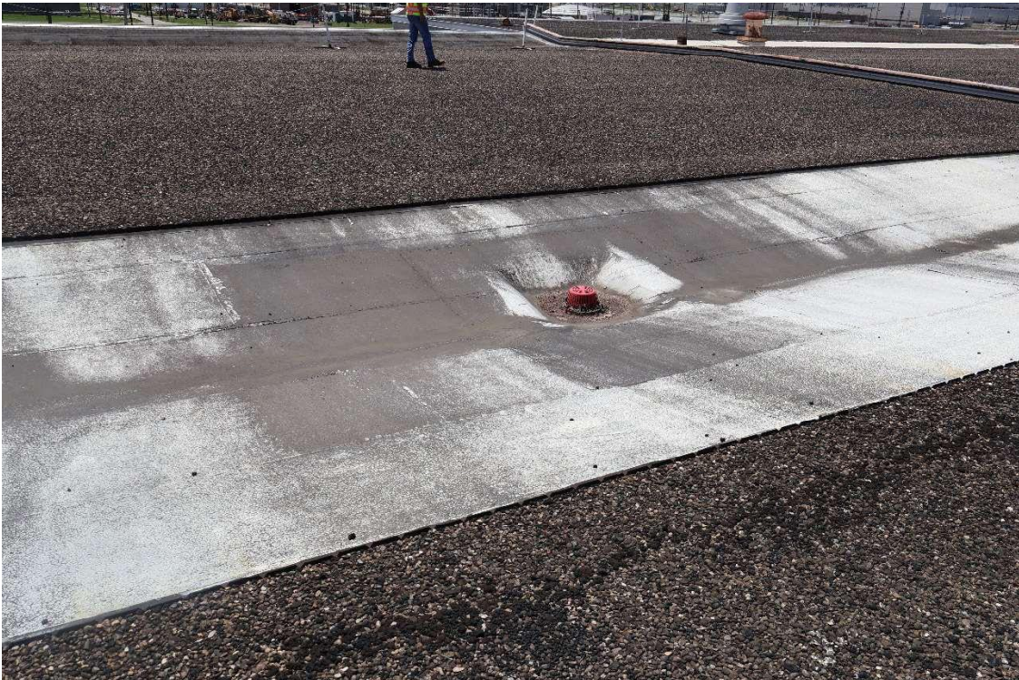
Main High roof – typical drain in valley
