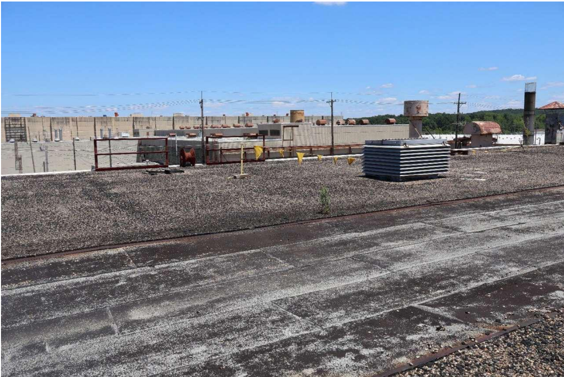
Main High roof – More vegetation on North side
