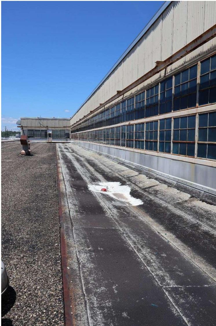
Main Low roof – Valleys near the main high roof
