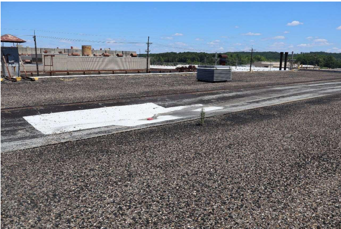
Main High roof – Vegetation on North side
