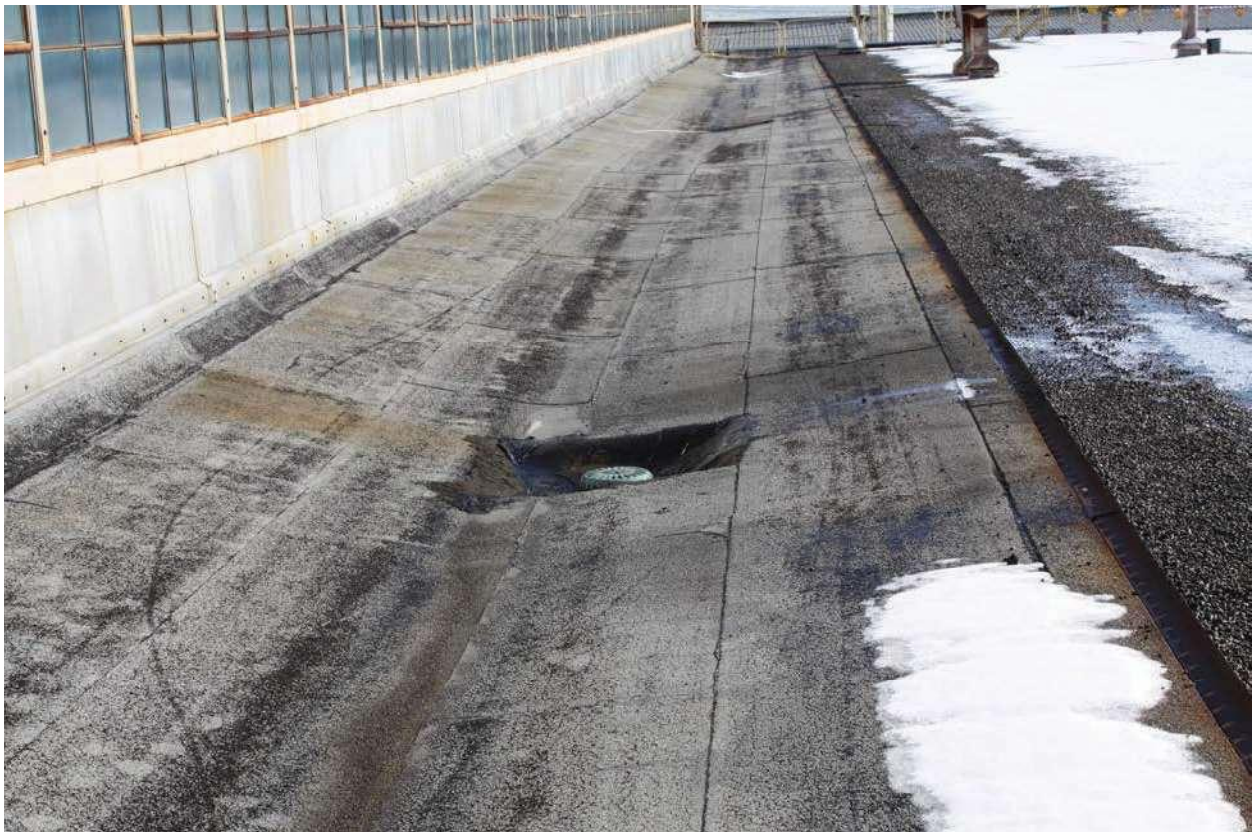
Looking East – Main Low Roof
