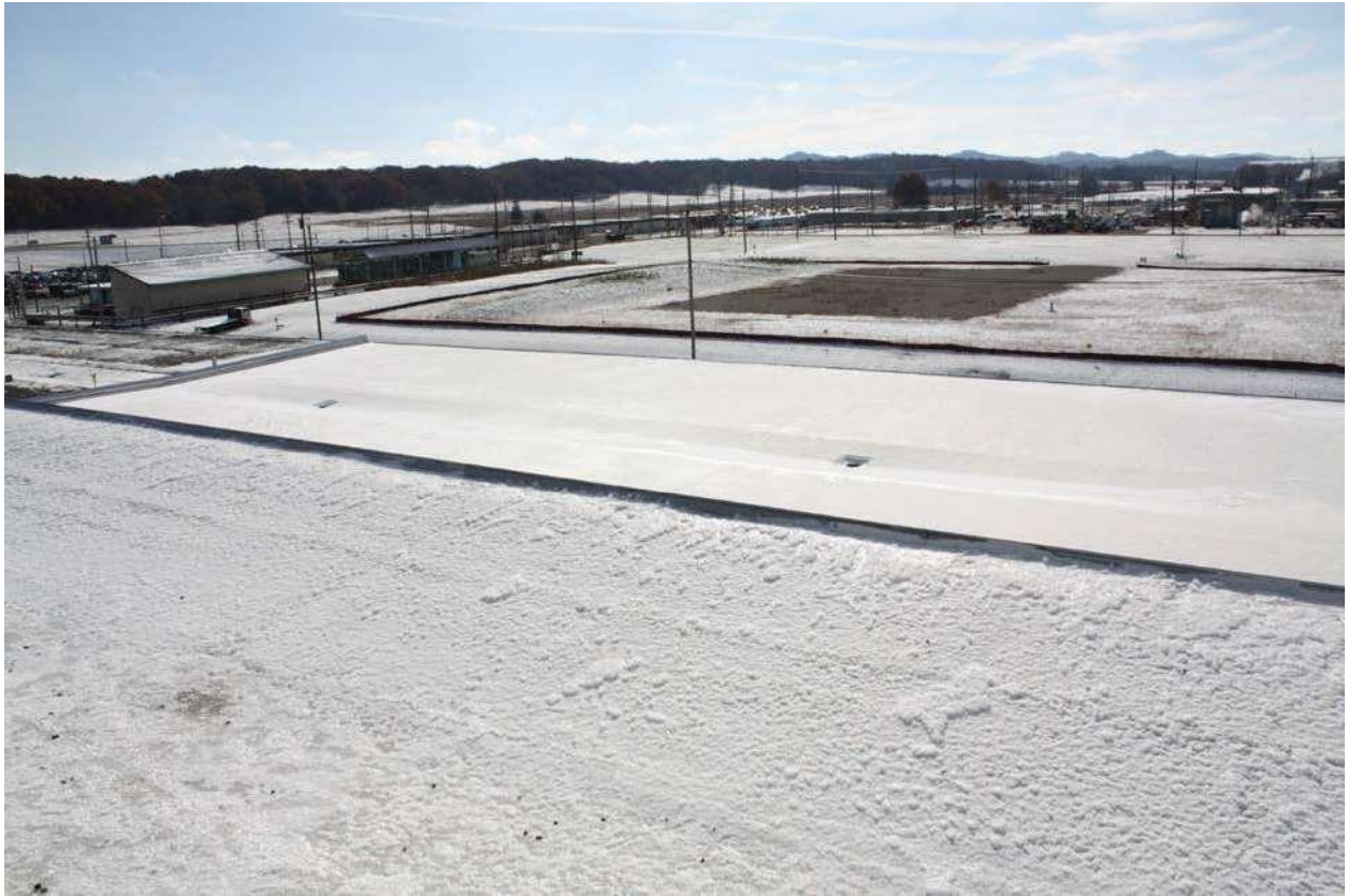
Looking Southeast from Highbay at New TPO on Main Low Roof
