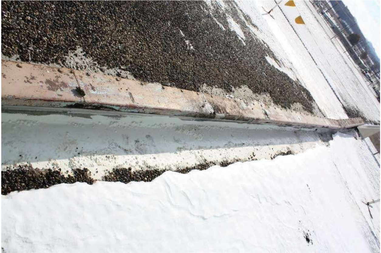
Past Repair of Expansion Joint on Highbay Roof
