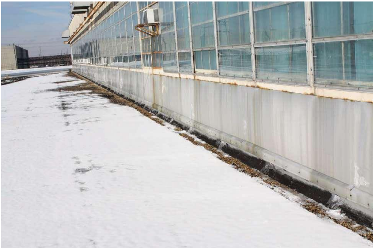
Looking West on Main Low Roof
