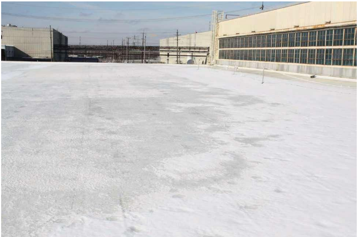
Looking West – New TPO on Main Low Roof
