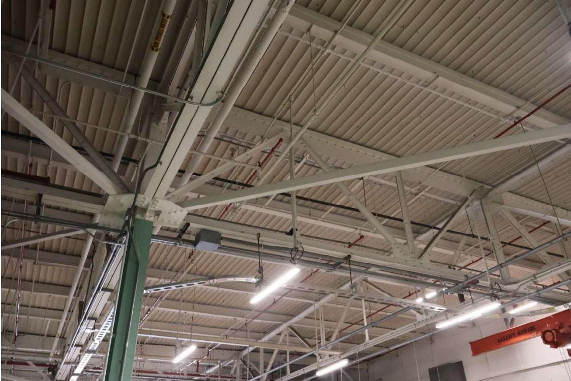
Near column B18
