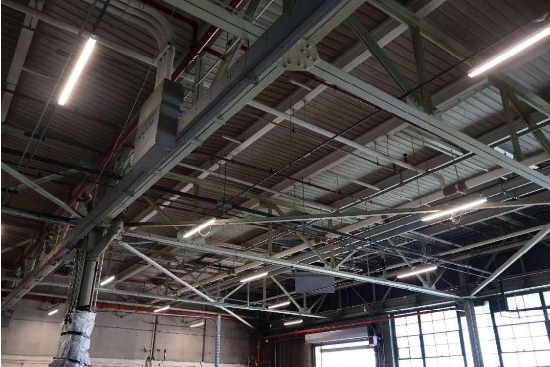
Near B15 in Stores Area
