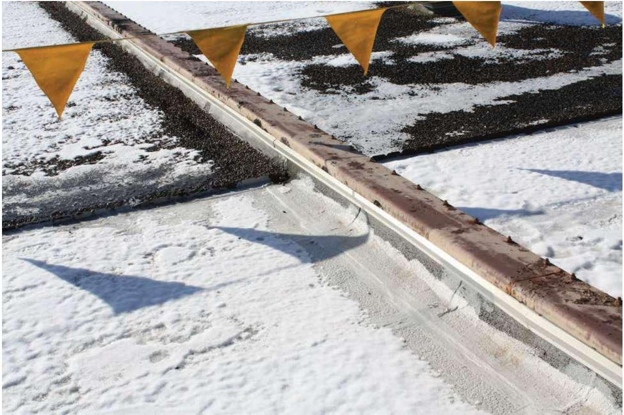
Main Low Roof – Repair at Expansion Joint
